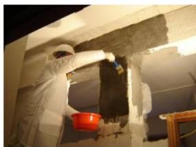
The new developed materials can be used, even, for structural renovation and consolidation of buildings in the warmer areas of the Mediterranean basin. Besides, new FRG composites, with permeability behaviour, are eco-friendly with the architectural heritage.
